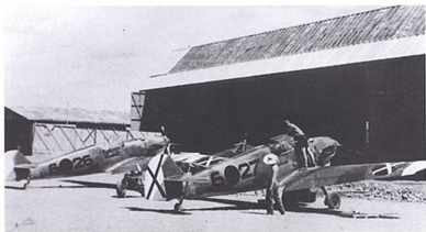
ABOVE: A pair of Bf 109 B-2s in service with Jagdgruppe 88 during the autumn of 1937. The first Messerschmitts were delivered in overall pale grey (65) finish but later this was overpainted with irregular medium green (62) stripes, with the undersides painted in pale blue (65).
