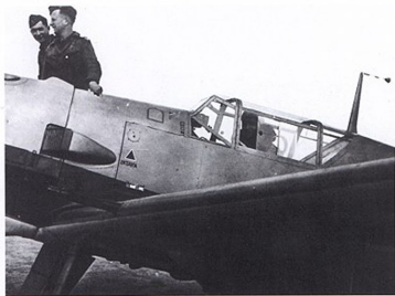
ABOVE: This close-up of a Bf 109 E shows the red oil filler triangle positioned behind the carburetor air intake with the inscription "INTAVA" underneath. The pilot has slid back the glass panel in his canopy.
