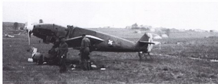
LEFT: The same Bf 109 B-1 as shown above, later on in the war after it had been converted to a B-2 variant, with a two bladed variable pitch metal propeller. At this time the aircraft had also been re-painted in medium green (62) and the code 605 re-applied in the new fatter style numbers.
