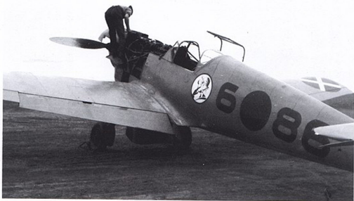
ABOVE: A mechanic working on the last Bf 109 D-1 to be sent to Spain coded 6086. The aircraft was delivered to 1J/88 which had just adopted the 'Holzauge' emblem.
